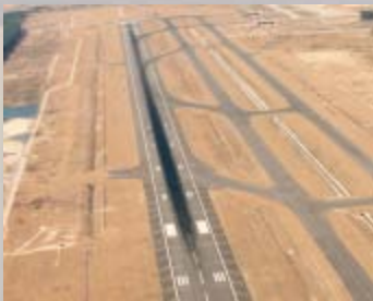
10,000 ft. long, Runway 09/27 went operational in 1987.
