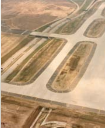
Bridging the gap: New taxiways spanning the airport approach roads in May 1987.
